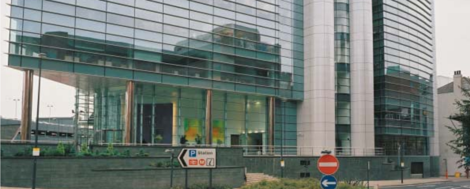
Leeds, Princes Exchange
